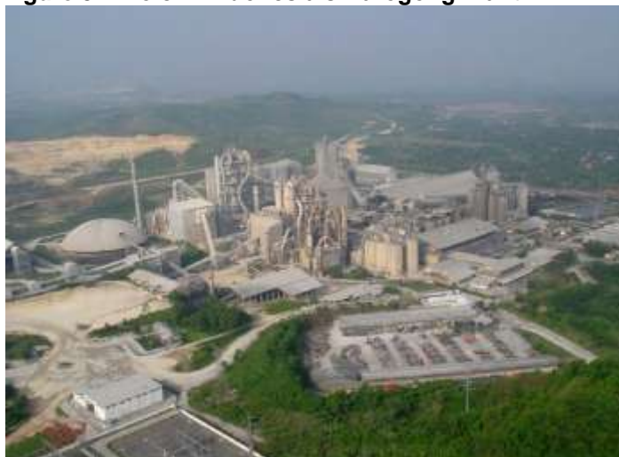
Figure 31: Holcim Indonesia's Narogong Plant
