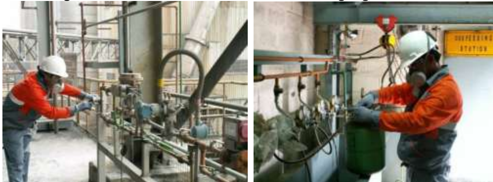
Figure 33: ODS destruction at the Holcim Narogong cement kiln
