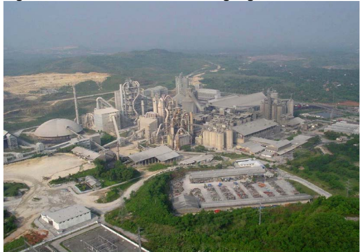
Figure 12: Holcim Indonesia's Narogong Plant
