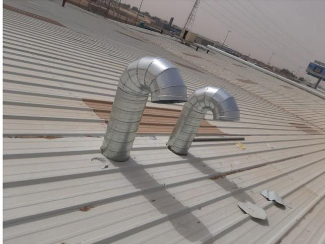
*Figure 9. Exhaust vent on the roof of the production line area.*
