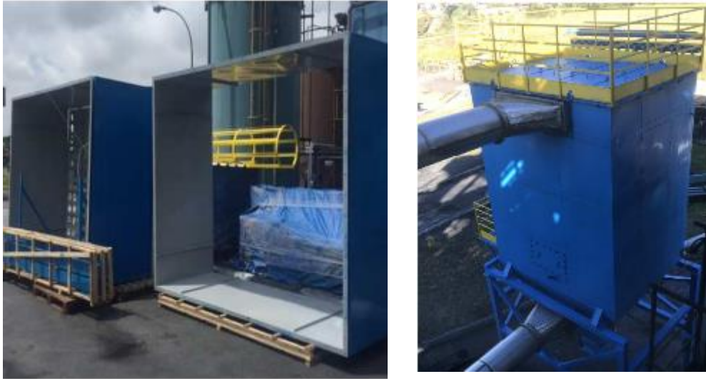
Figure 11 – Bag filter: before and after installation.
