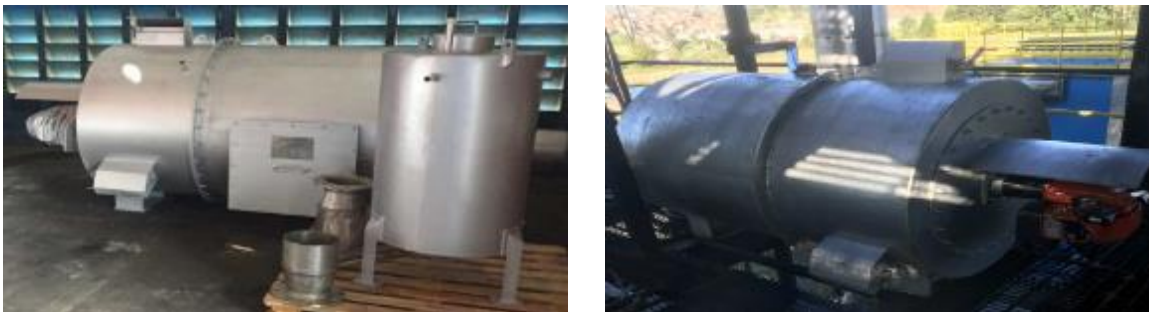
Figure 12 – Hot gas generation system before and after installation.
