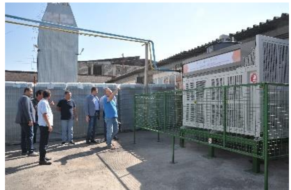
Fig. 14 Training course in class and on site
