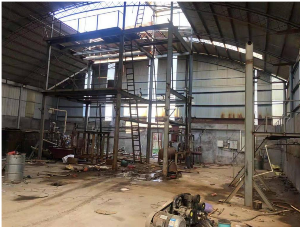
Production site after dismantling and removal of production equipment
