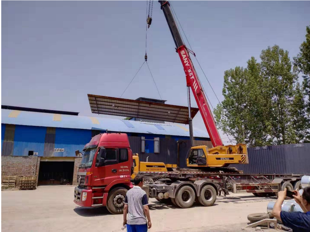
Production site being demolished
