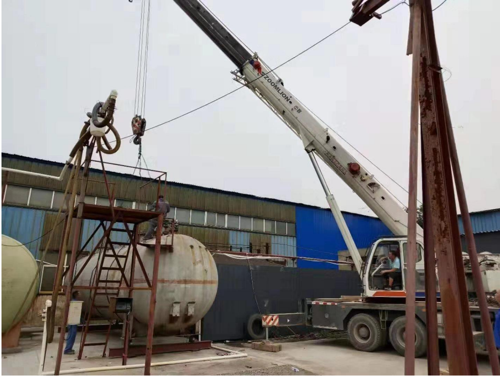
Dismantling of production equipment
