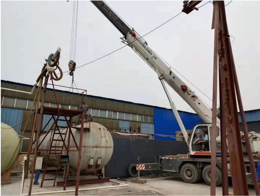
Dismantling of production equipment
