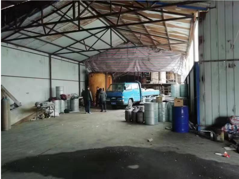
Dismantling of the production line
