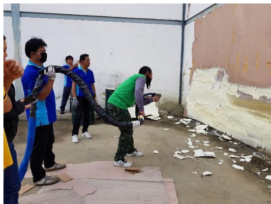
Fig. 3 Field Demonstration of HFO blown foam (HFO-1233zd(E)) at BIT
