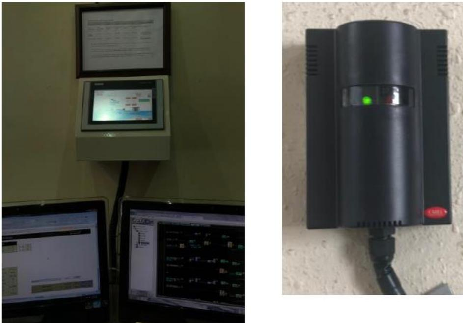
Figure 13: Control Alarm Panel and R-290 Sensors
