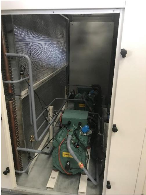
Figure 9: R-290 Unit with Semi-Hermetic Compressor
