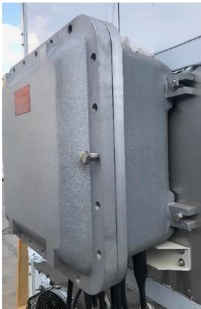
Figure 11: NEMA 7 Electrical Panel Upgrade
