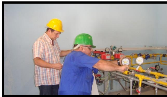
Picture 8. Storage area for cylinders (Source: OTOZ).
