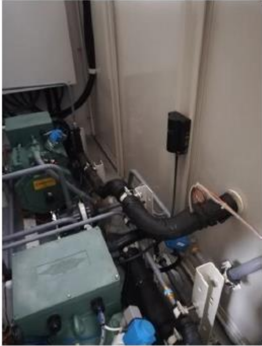
Figure 10: R-290 Leak Sensor
