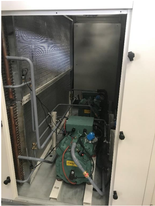
Figure 9: R-290 Unit with Semi-Hermetic Compressor
