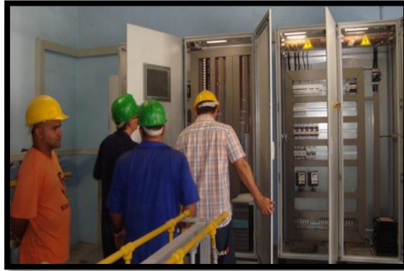
Picture 7. Assembly of supply lines (Source: OTOZ)
