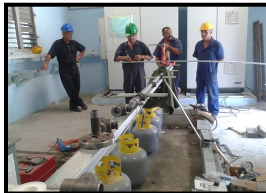
Picture 5. Construction of the ODS disposal plant (Source: OTOZ).
