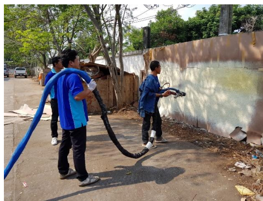
Fig. 4 Field Demonstration of HFO blown foam (HFO-1336mzz(Z)) at BIT
