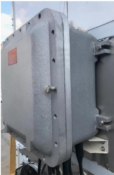
Figure 11: NEMA 7 Electrical Panel Upgrade
