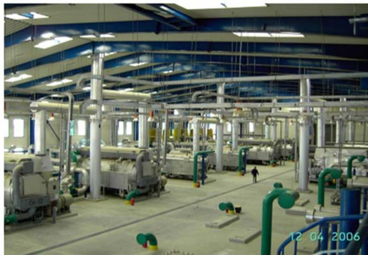
Figure 2.5: DC plant with 8000 TR gas fired absorption chiller/heaters.
