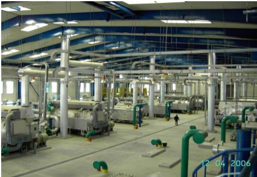
**Figure 1.1: DC plant with 8000 TR gas fired absorption chiller/heaters.**
