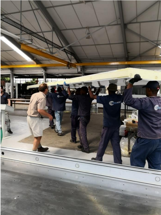
Foamed panel manual unloading
