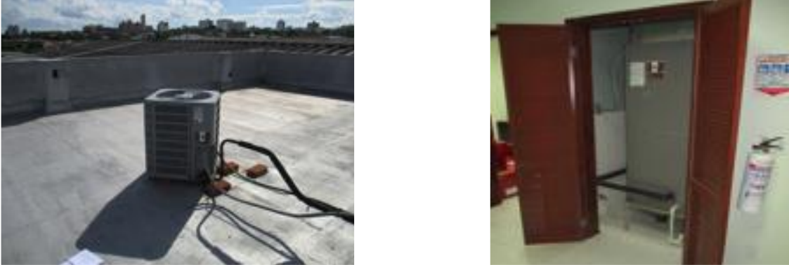
Figure 3: Typical installation example of ducted split DACS; condensing unit (left) and AHU (right)
