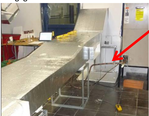
Figure 73: Test arrangement with return duct inlet indicated with red arrow
