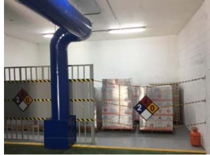
Figure 5.9: Civil and technical adaptations to the exterior and interior of the storage room (ventilation system)
