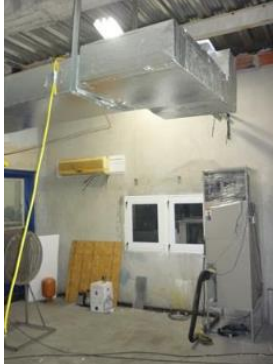
Figure 5.1: Mock elevated AHU and associated single ducting
