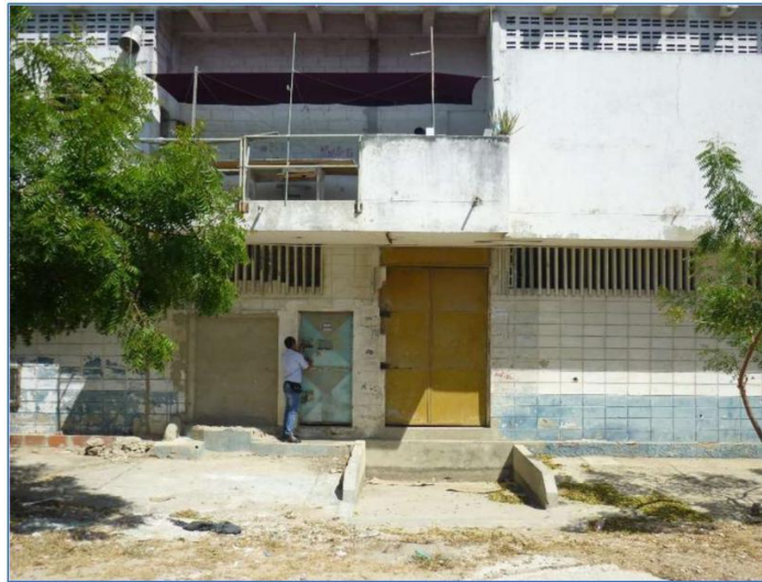
Fig. 1. External Storage of R290
