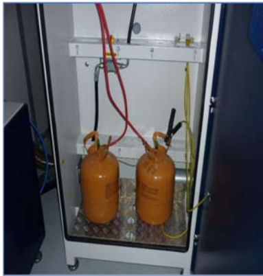
Figure 4.19: Storage compartment of R290 refrigerant gas (capacity: 4 cylinders, 5.5 kg each); charge and leak test equipment.
