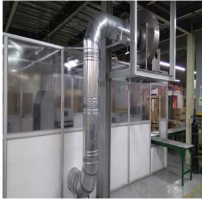
Figure 4.19: Storage compartment of R290 refrigerant gas (capacity: 4 cylinders, 5.5 kg each); charge and leak test equipment.
