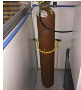
Figure 5.11: Installation of a pedestal with a safety chain to prevent the fall of the Helium cylinder.
