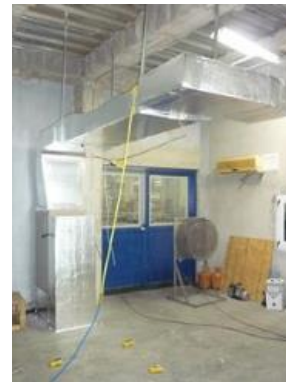
Figure 113: Mock elevated AHU and associated single ducting and surrounding test area
