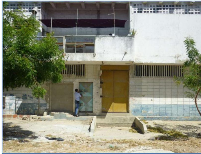
Fig. 1. External Storage of R290
