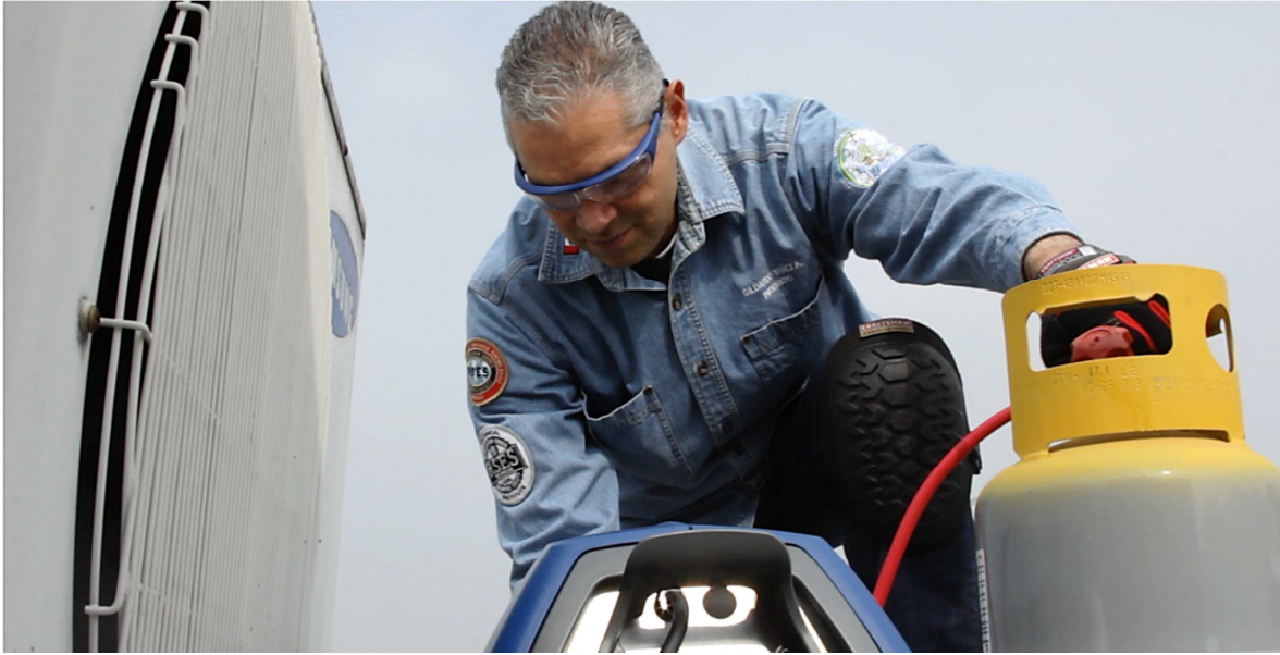
Figure 6 ODS recovery by Mexican servicing technicians
