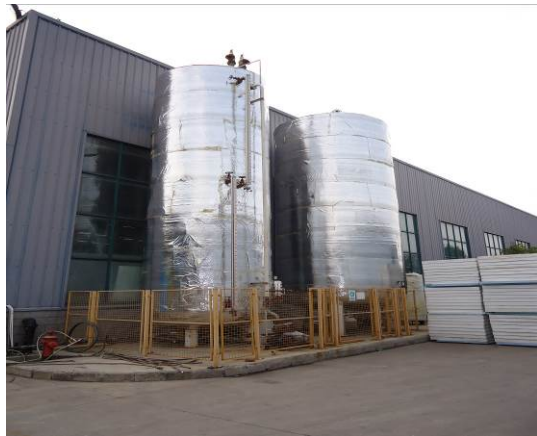
Blowing agent tank and diaphragm pump metering system
