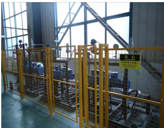
Blowing agent tank and diaphragm pump metering system
