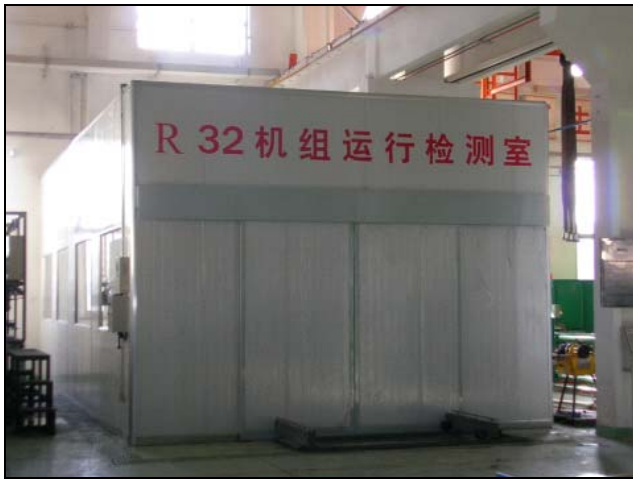
R32 products operating testing room
