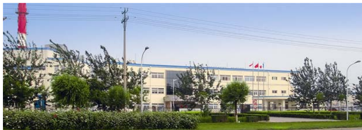
Figure 8: Hejia Velia facilities
